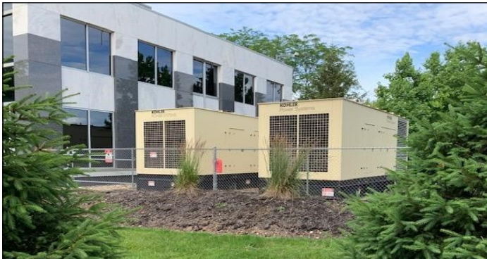
Kohler generators—North Wing
