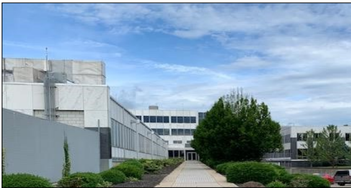
Westward view of VTP—CyrusOne Data and building entrance
